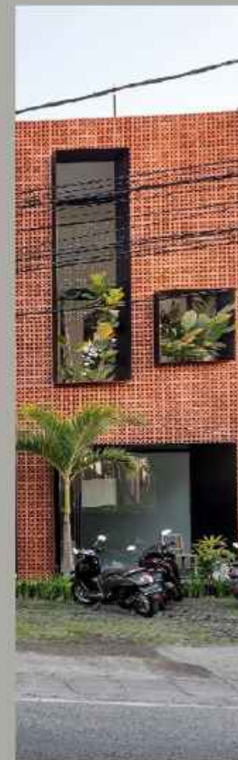
TERAS Soho Style Apartments
