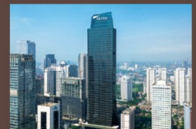
Astra Office Tower
