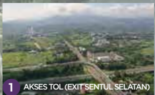
1 AKSES TOL (EXIT SENTUL SELATAN)
