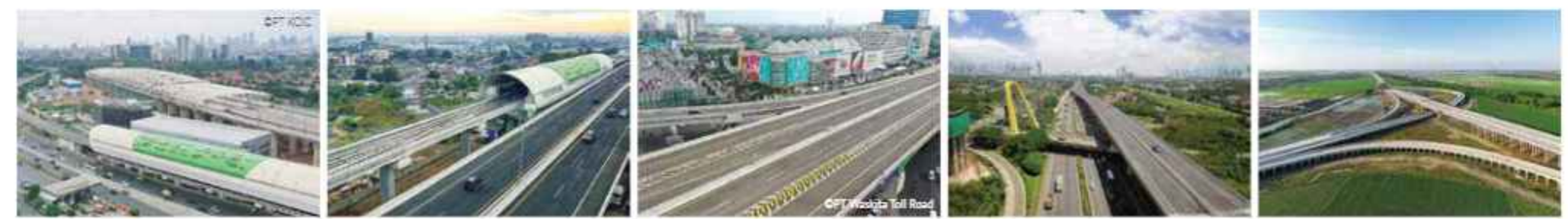
HALIM FAST TRAIN STATION | LRT STATION - BEKASI TIMUR | BECAKAYU TOLL | JAKARTA-CIKAMPEK ELEVATED TOLL | JORR 2
