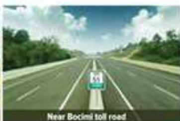
Near Bocimi toll road
